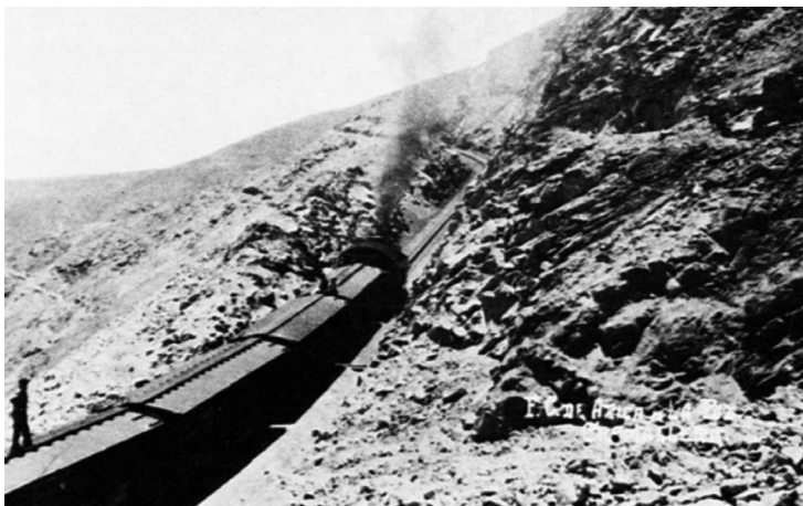
Figura 67: Foto histórica del Ferrocarril de Arica a La Paz en funcionamiento. Figure 67: Historical picture of the Arica - La Paz railway in operation.
